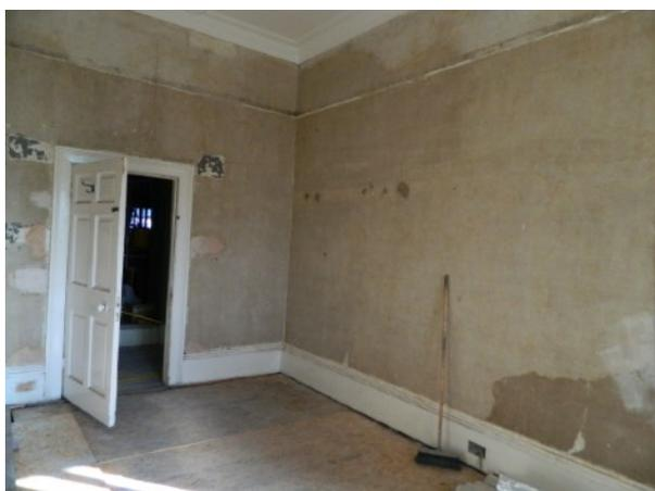
Work is currently ongoing to re-lay the floors on the third storey and repair plasterwork in the State Room, a delicate operation that involves fixing a layer of mesh to the damaged sections, over which new plaster can be laid. The two rooms that will become the silver galleries have been stripped out ready for painting, while in the basement a new kitchen range will be built in situ over the next few weeks.
